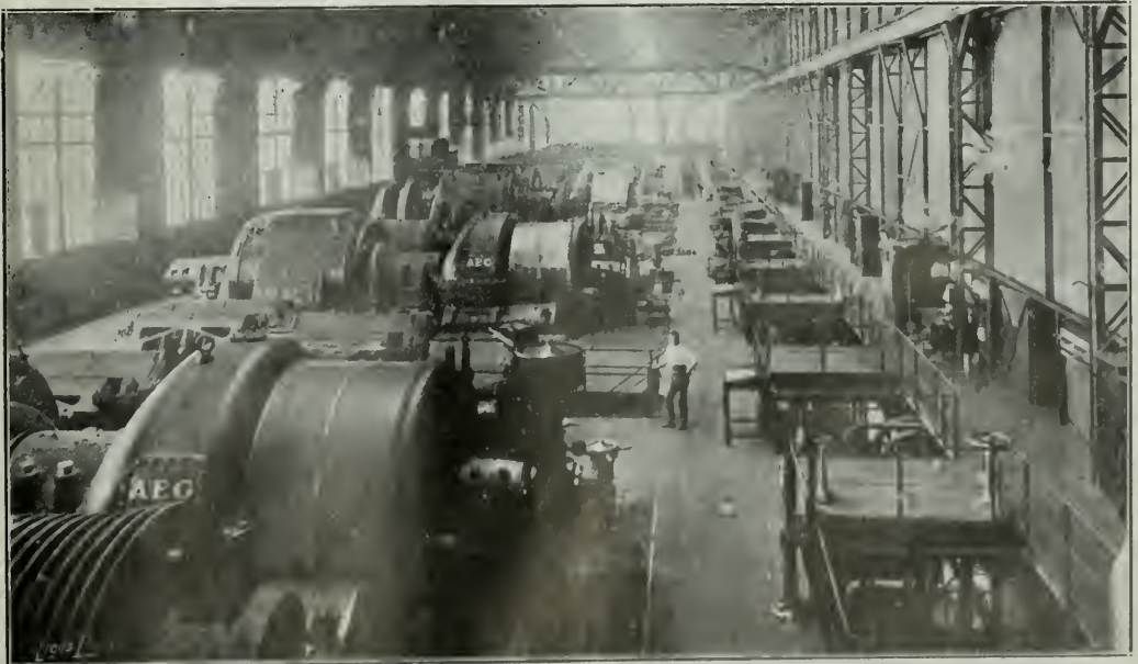
ROSHERVALE POWER STATION INTERIOR
